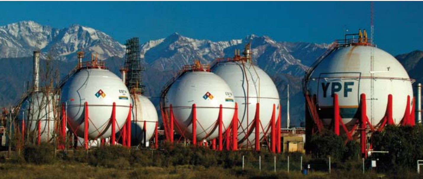
The Lujan de Cuyo refinery (Argentina), with the Andes in the background.
