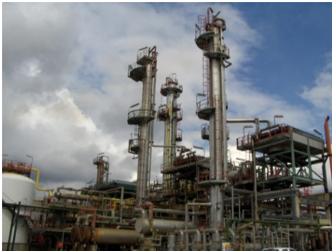
SOUR WATER AND SULPHUR RECOVERY UNITS MODIFICATIONS
