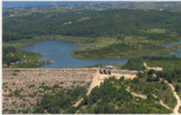
Land Custody Agreement for the Gaià Reservoir, Spain.
